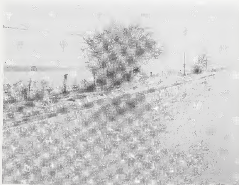
Flooding Along State Route 714 February 3, 1982
